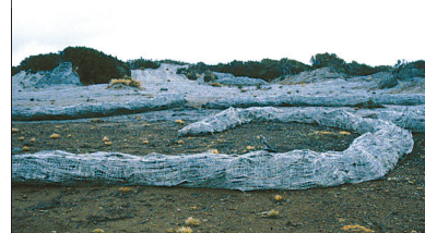
Jute and slash work are used to stabilise the degraded Lake Ada lunette, Central Plateau.
