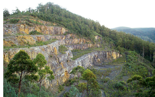
Lune River Quarry showing the results of the rehabilitation program, June 2001. Rehabilitation successfully stabilised the quarry benches and resulted in marked improvements in the water quality and ecology of the nearby Exit Cave area.
