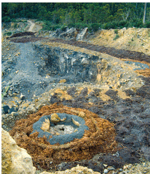
A filter bund surrounding a cave entrance exposed by quarrying. The filters were built from heavy limestone blocks, various grades of crushed limestone, geotextile filter membrane and various organic mulches such as sterile straw bales and Eucalyptus bark. These bunds prevented the ingress of bench sediments and applied topsoil to the cave system whilst vegetation was re-established.
