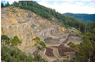
The Lune River limestone quarry following machine works for rehabilitation. Note the division of the benches into separate drainage cells, each feeding a vertical cave entrance or infiltration zone. This configuration attempted to reproduce the natural karst drainage systems of the Exit Cave area that were in existence prior to quarrying.
